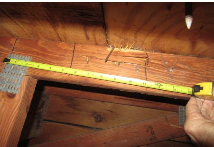
Nail location verified
