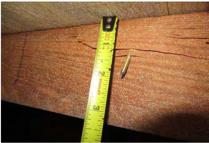
8d nails verified
