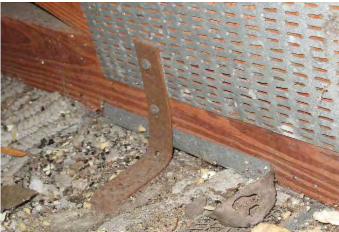
Single strap with 2 nails into the truss
