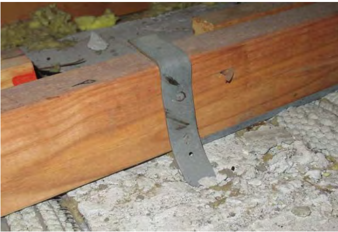
Single strap with 1 nail into the truss
