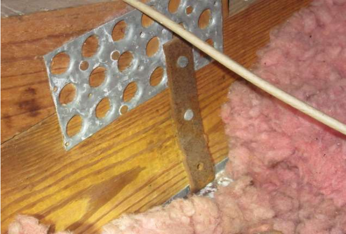
Single strap with 2 nails into the truss
