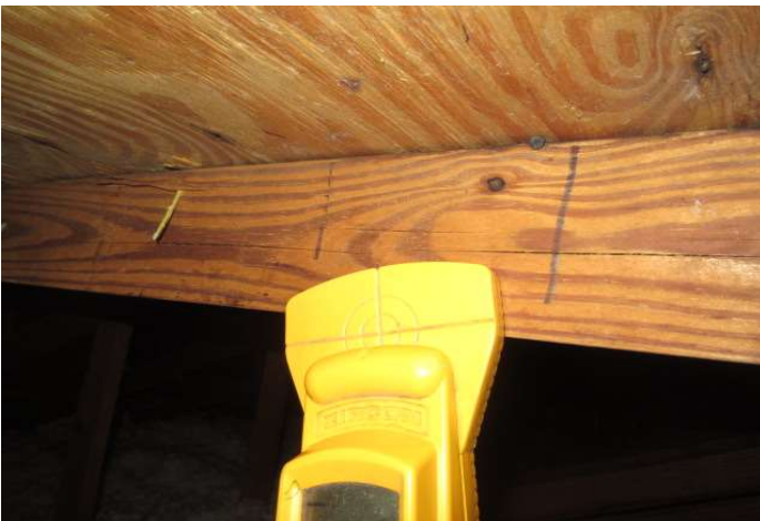
Nail location verified
