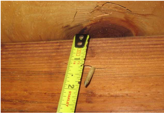
8d nails verified
