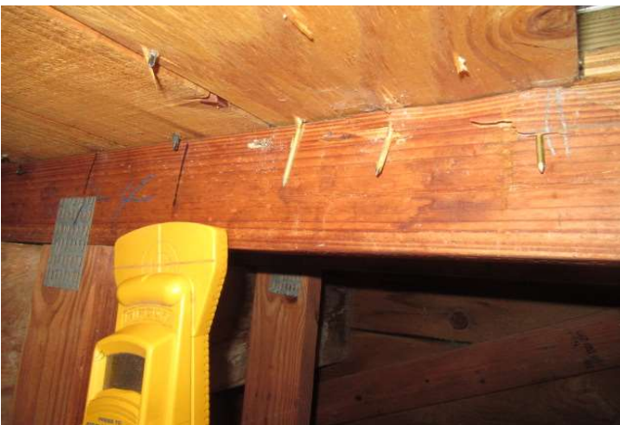
Nail location verified
