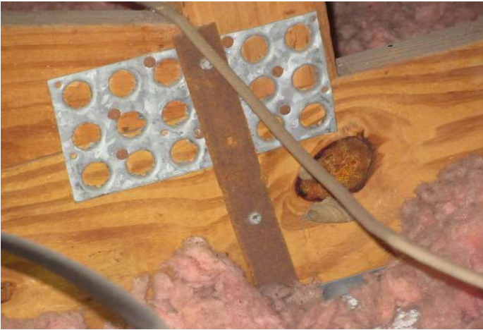
Single strap with 2 nails into the truss
