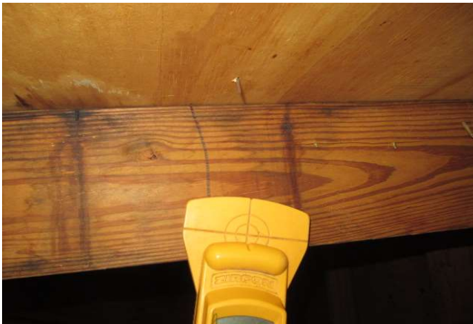
Nail location verified
