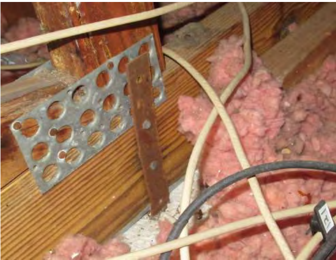
Single strap with 2 nails into the truss
