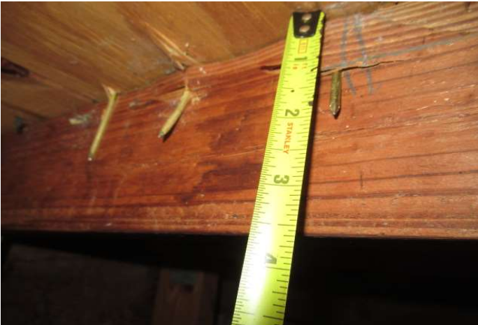
8d nails verified
