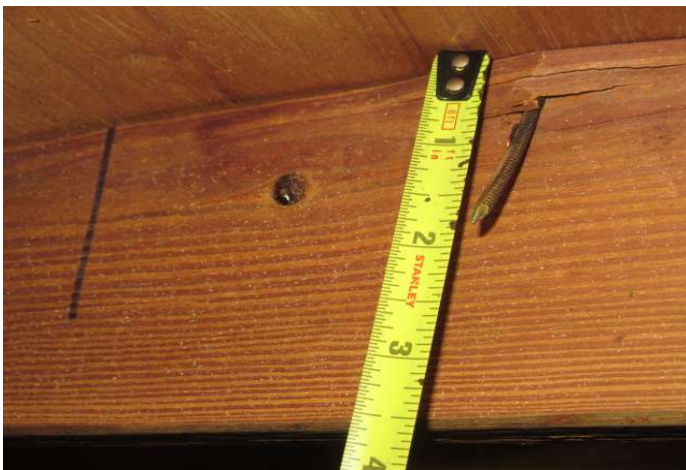
8d nails verified
