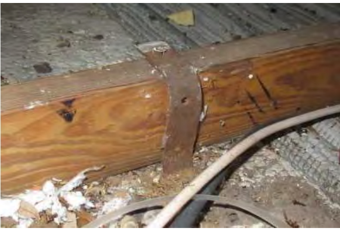
Single strap with 2 nails into the truss
