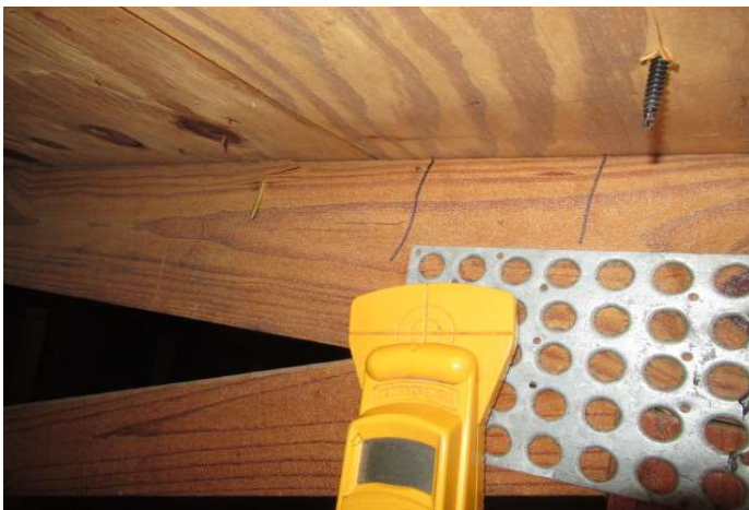
Nail location verified
