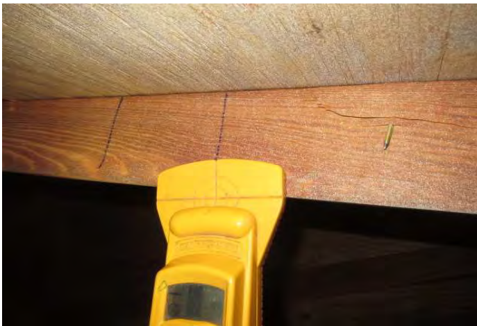
Nail location verified
