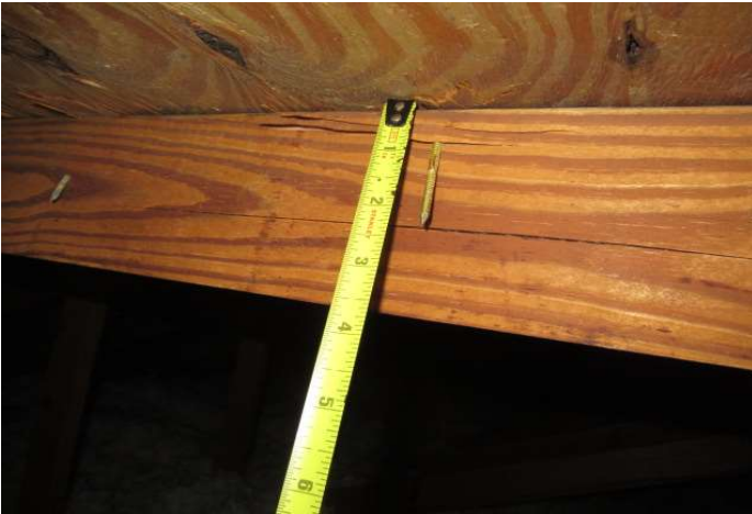
8d nails verified
