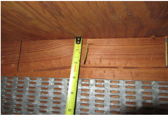
8d nails verified
