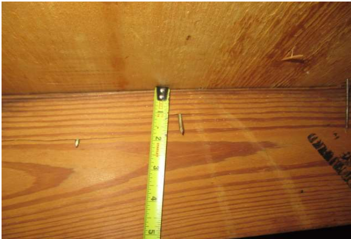
8d nails verified
