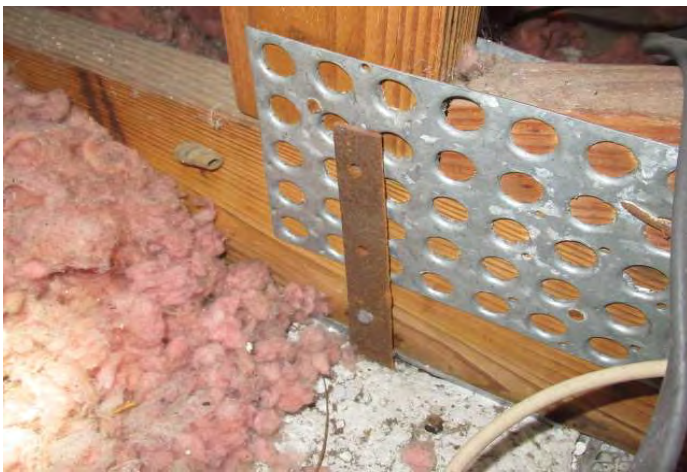
Single strap with 2 nails into the truss
