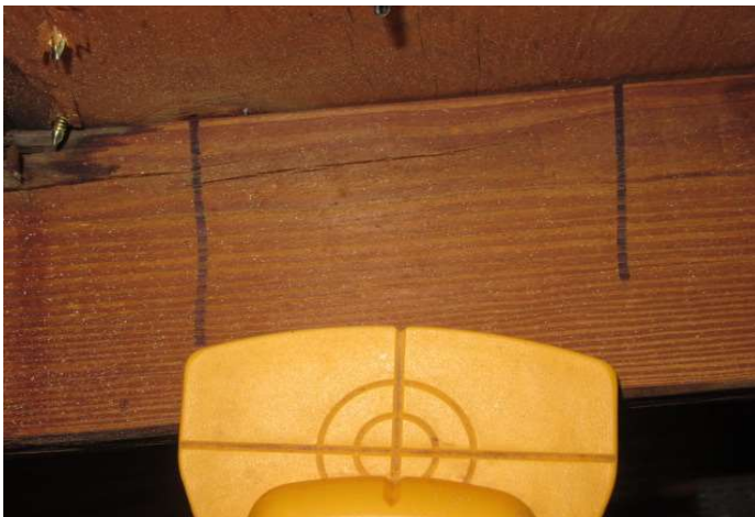
Nail location verified
