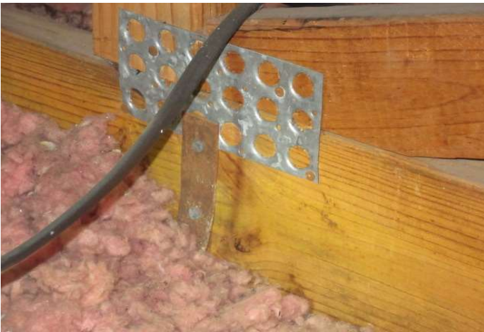
Single strap with 2 nails into the truss
