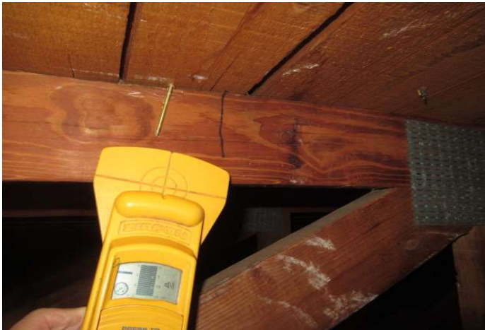
Nail location verified
