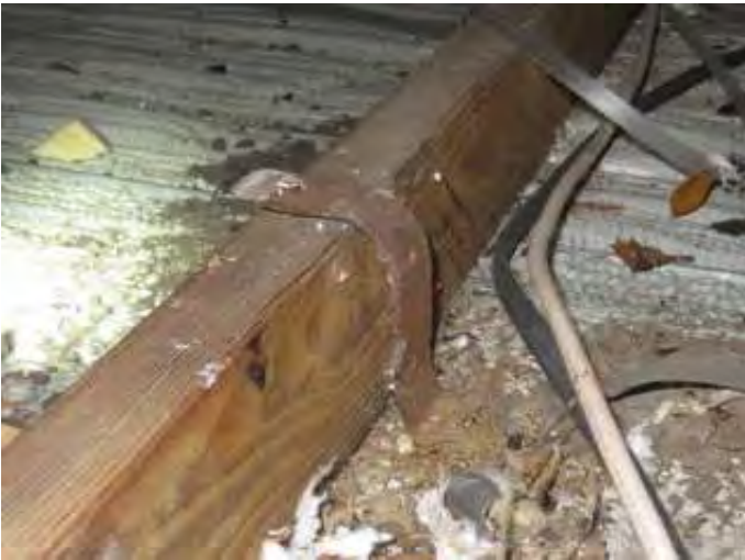
Single strap with 2 nails into the truss
