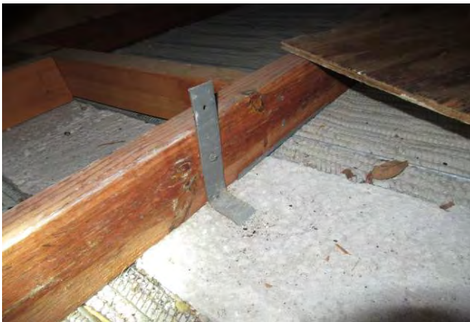
Single strap with 1 nail into the truss
